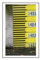
1402' above sea level which is the elevation of the spillway. These elevations are built into our dam "Inspection and Maintenance Plan" which is required by DEC. We use the elevations and current weather reports to tell us when the drains should be opened to lower the level of the lake. These gauges are important and should not be tampered with.
