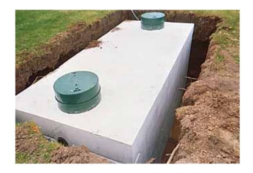
**Concrete 1,000 Gallon Septic Tank with Risers**
