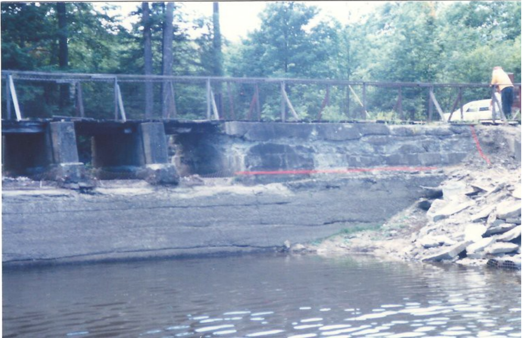
Upstream part of the dam to be removed for larger spillway
