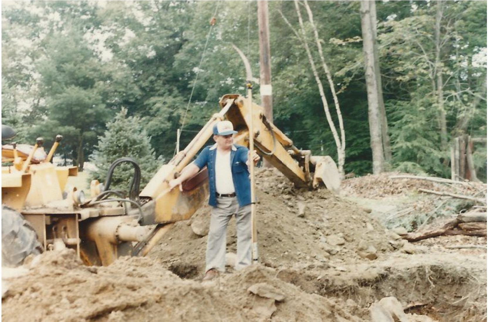
TEST HOLES WERE DUG TO DETERMINE DEPTH OF BEDROCK
