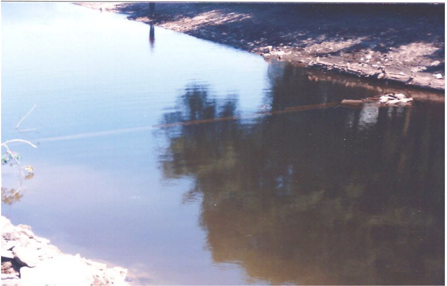
At this level, a wooden coffer dam which was constructed when the dam was built became visible
