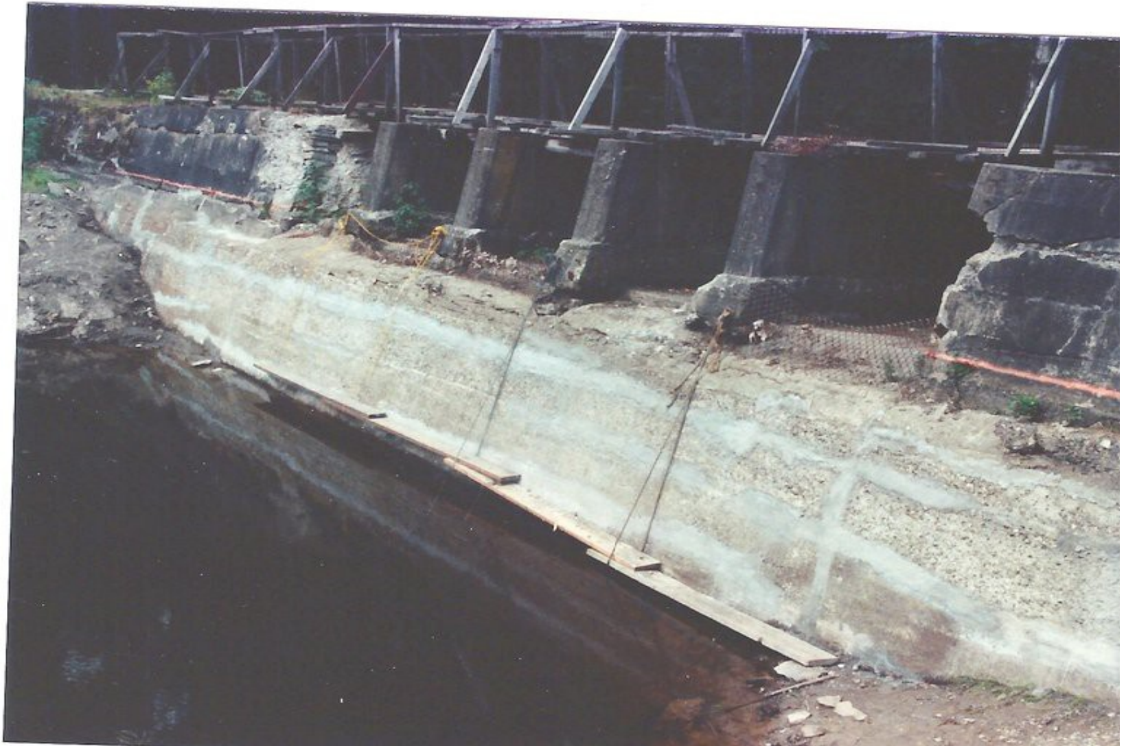
Cracks on the upstream face were patched with hydraulic cement
