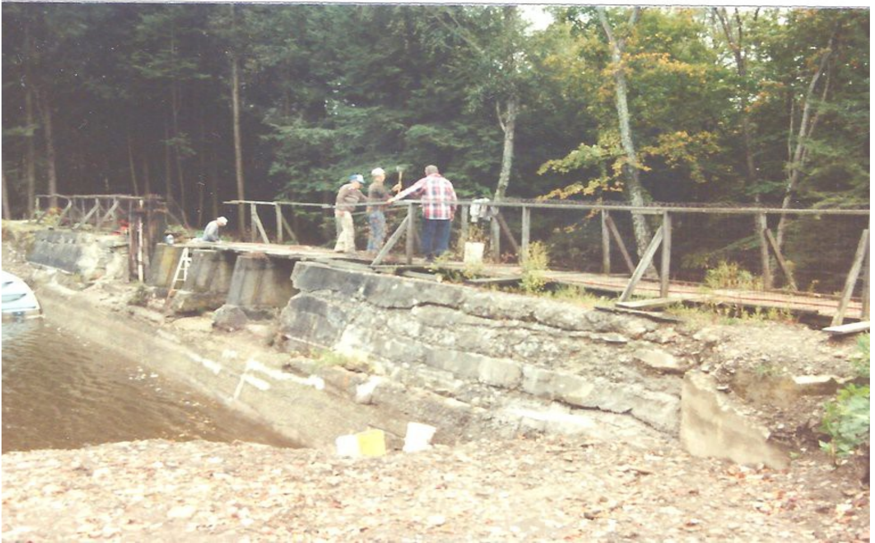
Again using association volunteers, the walkway was removed
