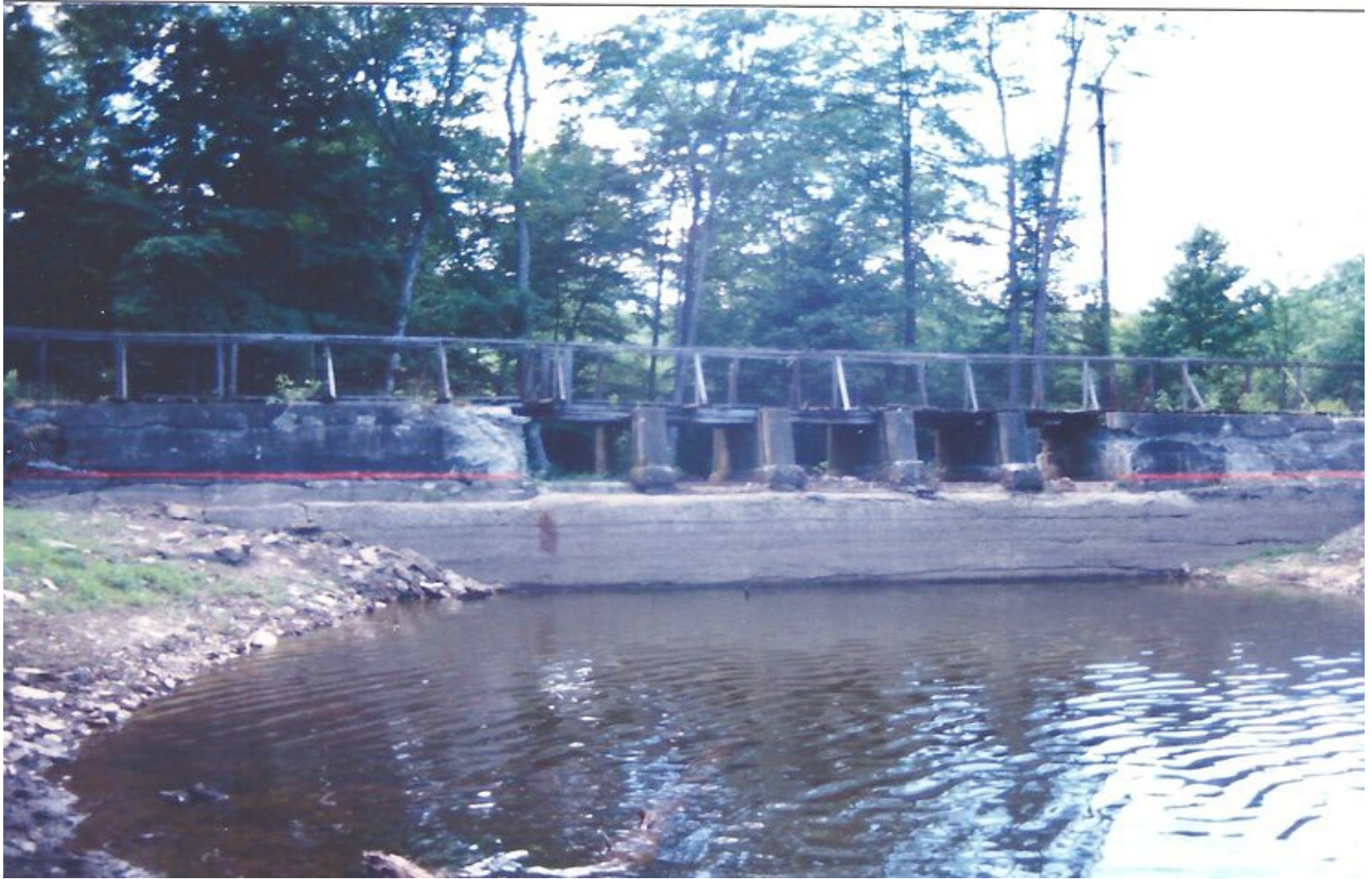
The Lake was lowered 7 feet which would allow us to inspect the upstream face of the dam
