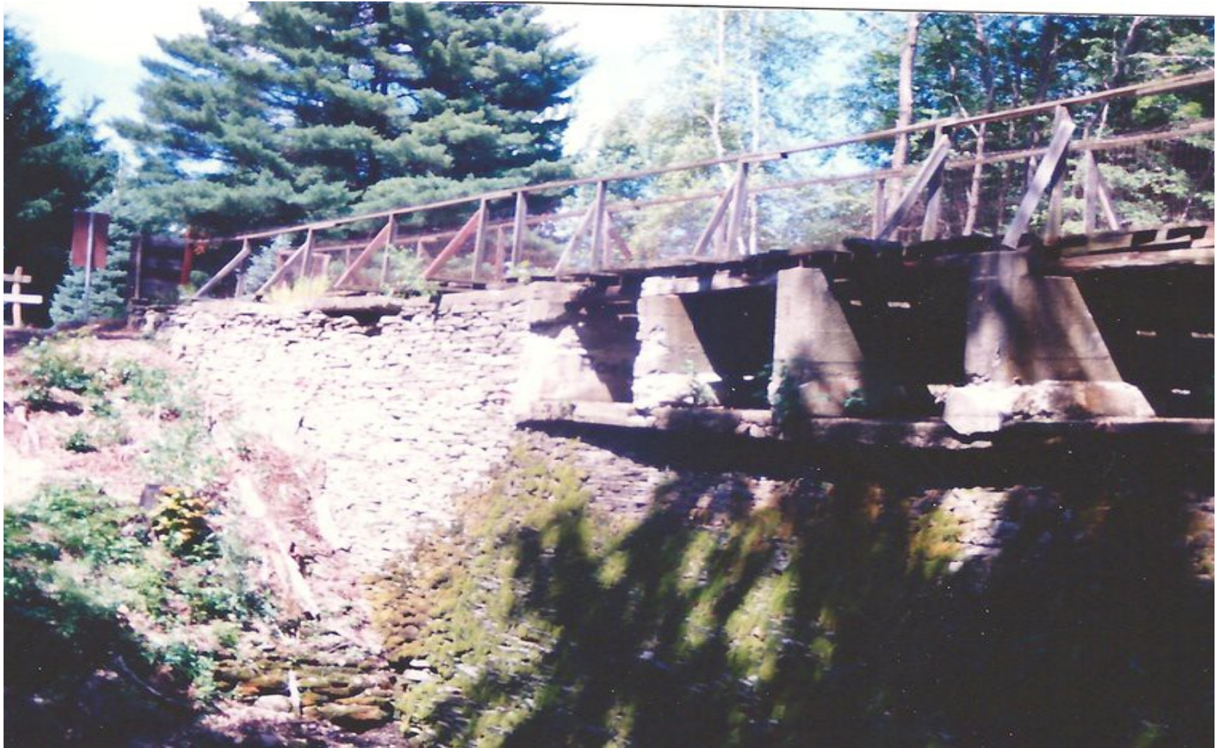
MISSING STONE AND DETERIORATED PIERS
