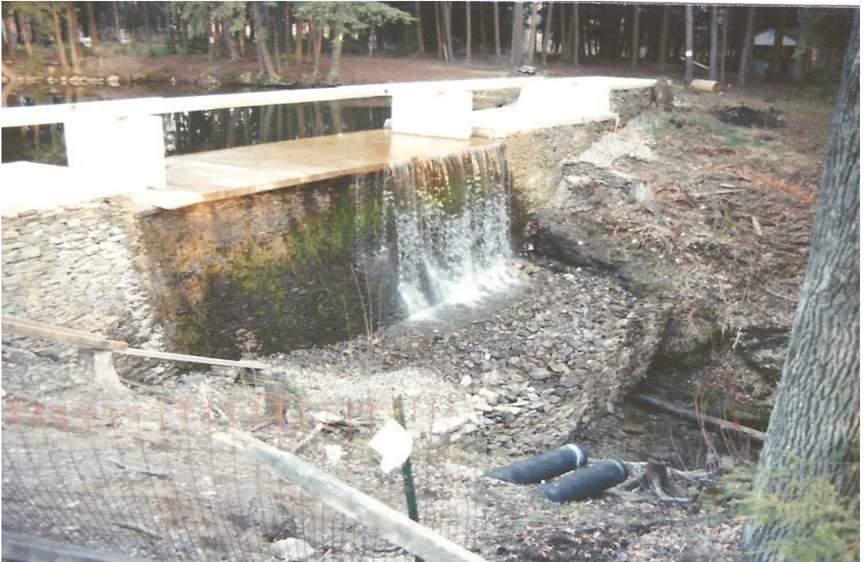
Work was started on the new walkway by Association Volunteers
