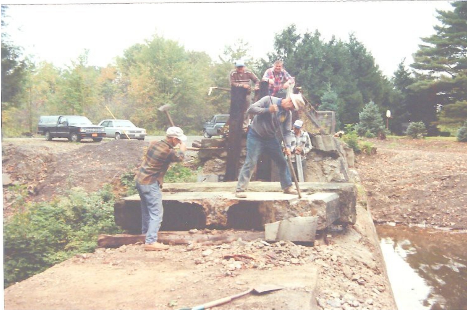
The piers were then removed
