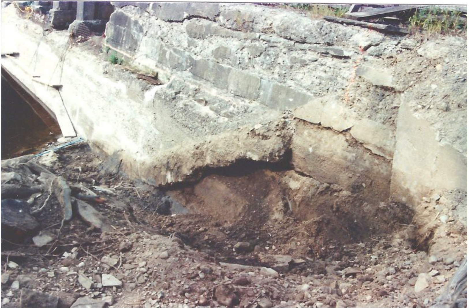
Larger sections were removed, formed and replaced
