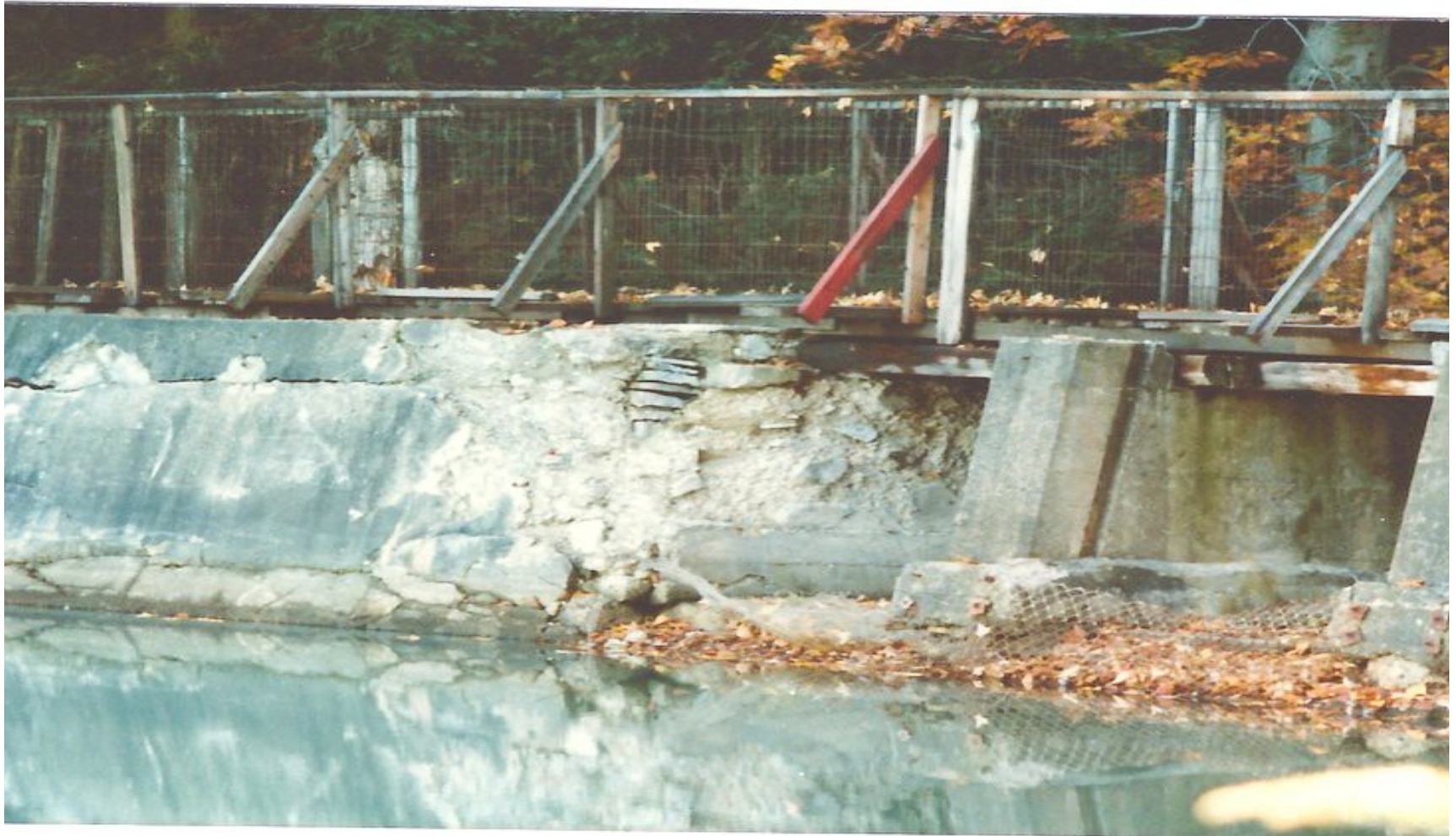
Upstream face of dam
