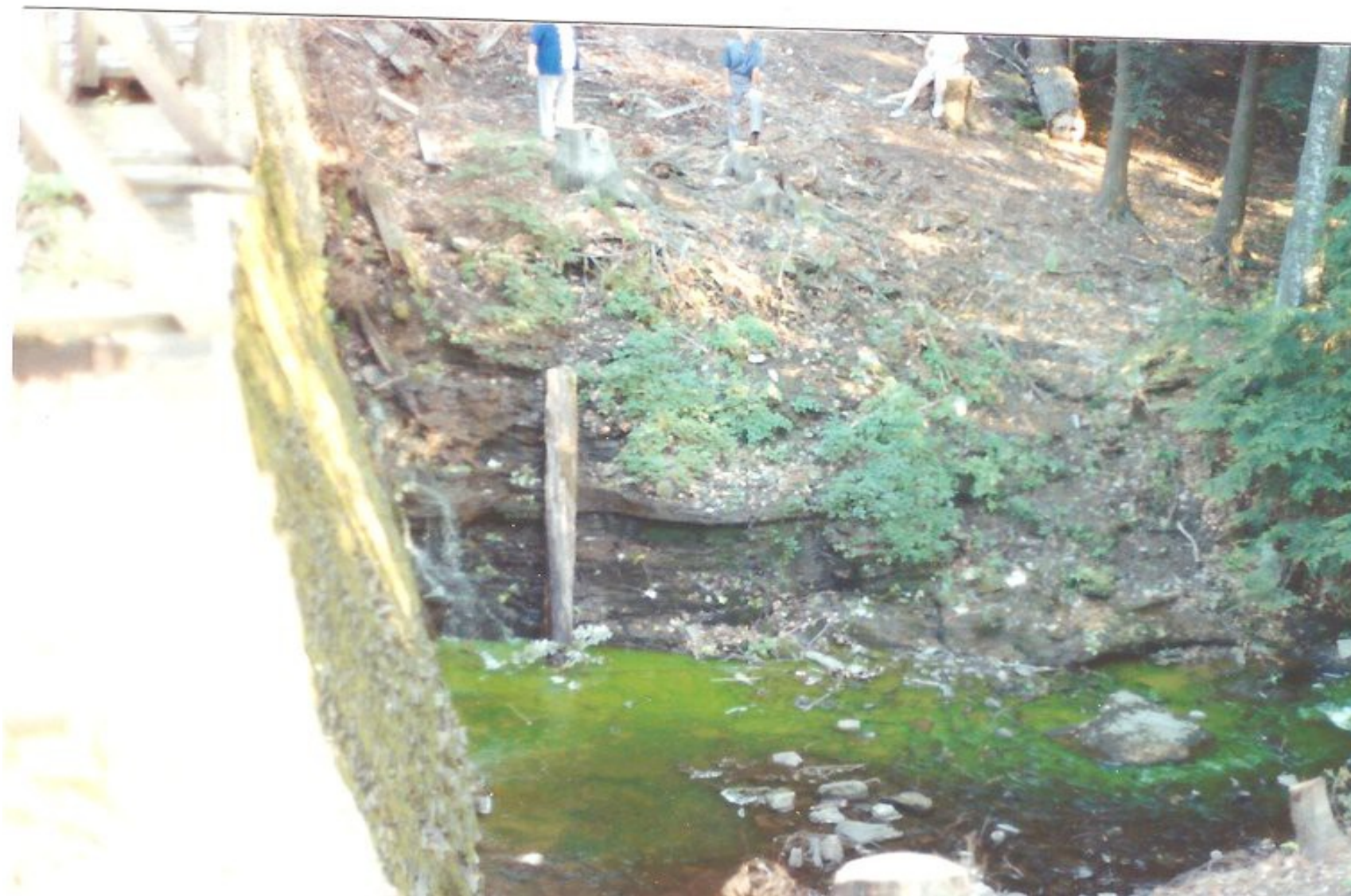
Dye was used to determine where the leakage was coming from
