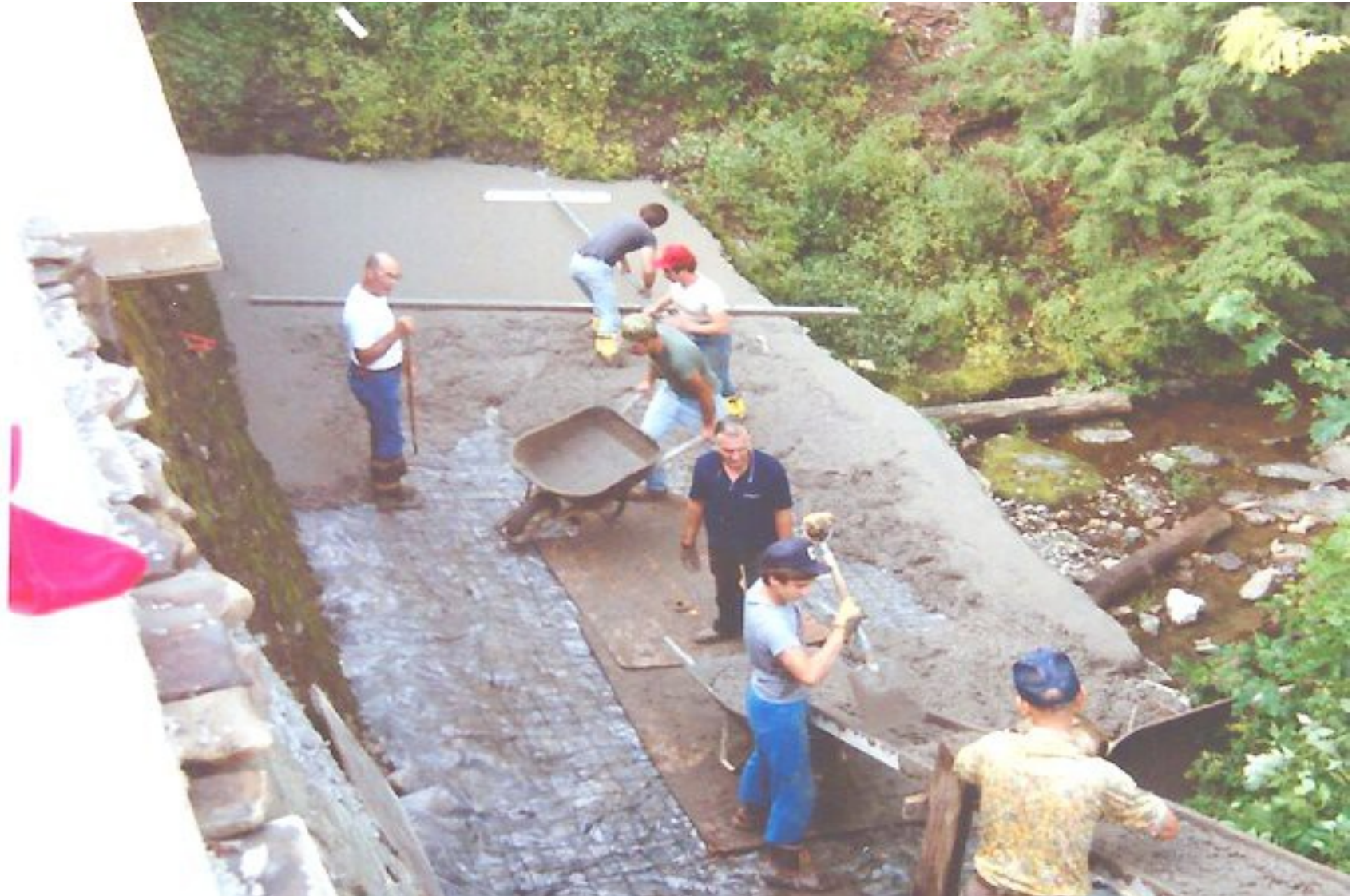
A concrete pad was poured by association members on the downstream buttress
