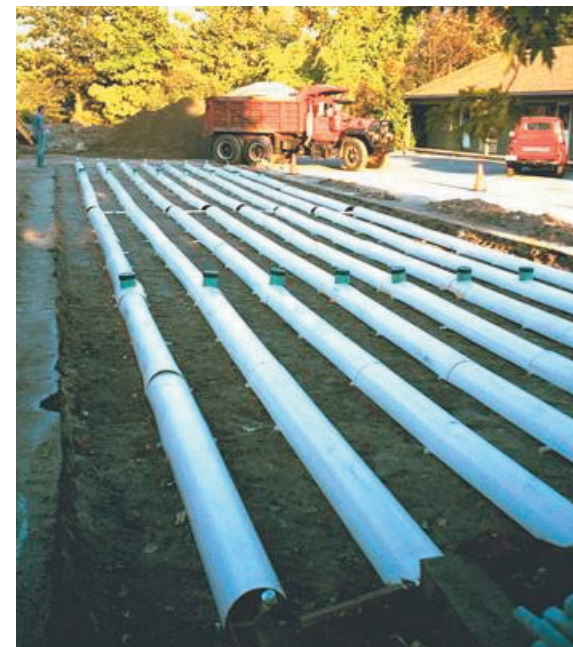
A shallow, narrow drainfield showing the outer PVC pipes that cover the pressure laterals. This drainfield serves a 2700 gallon-per-day restaurant and retail / office complex. These lines, located in a parking lot island, are ready to be covered with native backfill, and will be 12" below finish grade.
