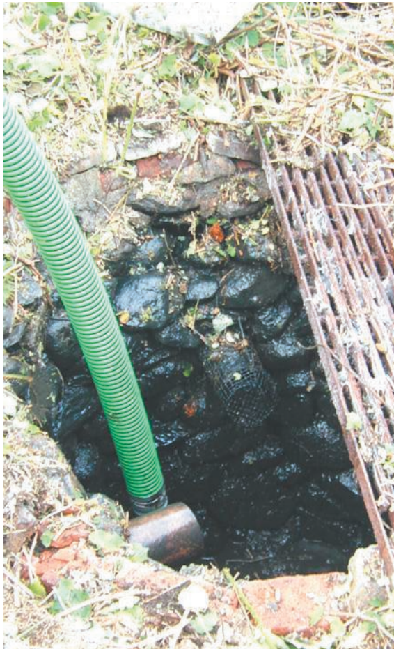
Dry fit rock cesspool being pumped. Because both solids and liquid effluent leach from cesspools, they are more likely to contaminate groundwater even where there is no obvious sign of surfacing effluent.
