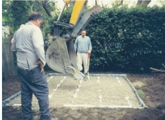
Installing a sand filter.
