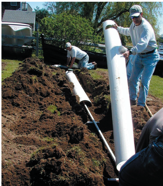
Installation of a shallow, narrow drainfield. Pressurized laterals (1" diameter PVC pipes) are shielded with 12" PVC pipe cut lengthwise, with at-grade inspection ports located at regular intervals. Shallow narrow drainfields take advantage of biochemically-active upper soil layers for microbial nutrient removal and plant uptake.
