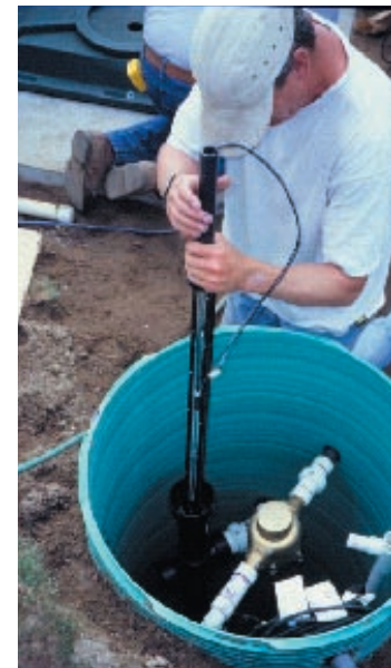
A pump chamber. This may also house recirculating valves, timers and other controls. The finished unit will have a green lid at the ground surface.
