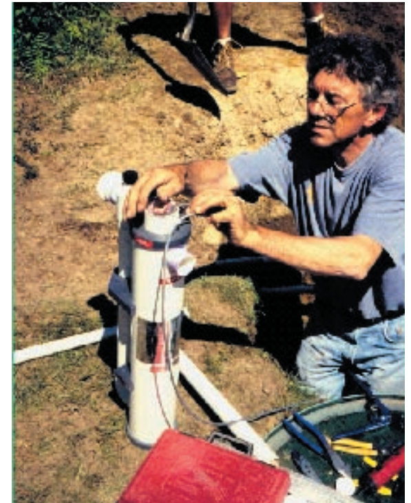
An ultraviolet light disinfection unit further reduces bacteria following the treatment unit. It typically fits into the pump chamber where treated effluent is pressure dosed to the drainfield for final dispersal.
